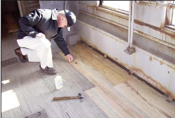
Bill Britt is finishing up the floor replacement.
